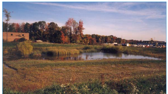
Water Quality Basin converted from a Detention Basin in Twinsburg, Ohio.
